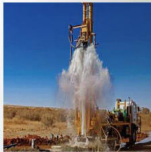
Water Well Drilling
