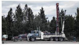
Water Well Drilling
